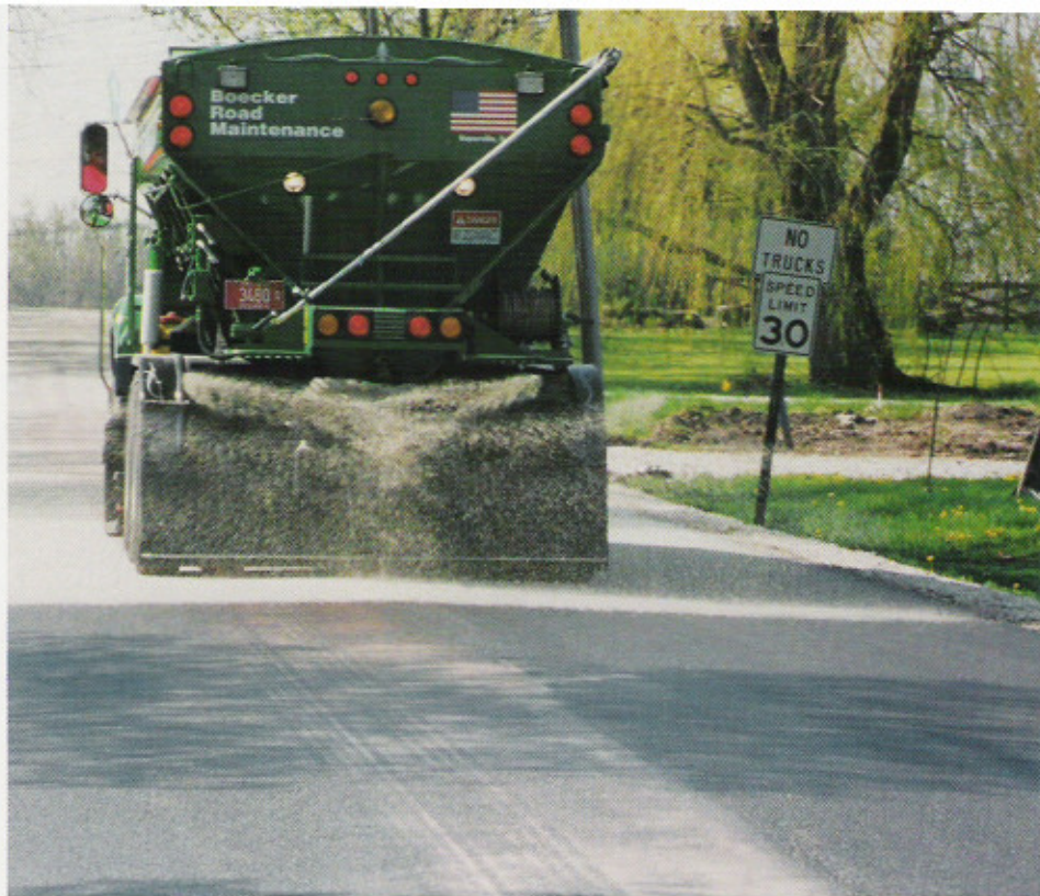
Sand trucks (above) are used to put down a layer of sand or limestone screenings. With the CRF the screenings are broomed (below) to evenly distribute the product over the surface and fill cracks and voids.
