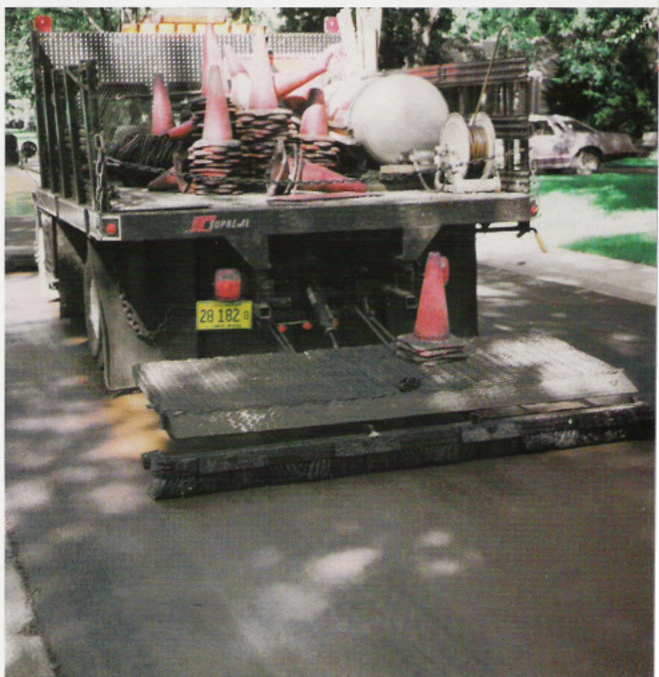
Sand trucks (above) are used to put down a layer of sand or limestone screenings. With the CRF the screenings are broomed (below) to evenly distribute the product over the surface and fill cracks and voids.
