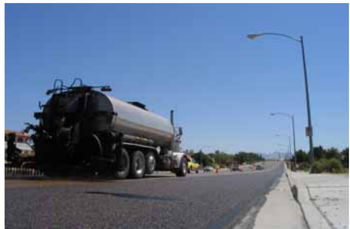
2. Reclamite® application by distributor truck. Product was diluted with water 1:1. Application rate was .13 gallons per square yard
