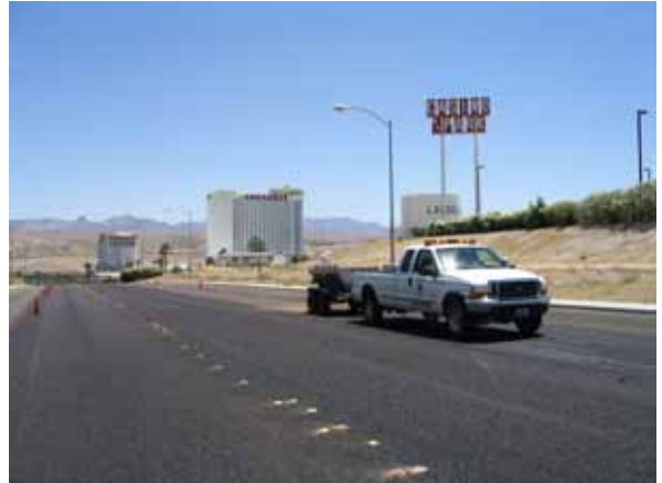
6. Sanding application by Clark County was applied at 2 lbs. sq. yard. (1 kg.sq. m.) A Spinner pull trailer was used.
