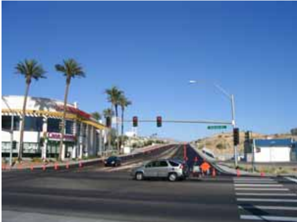
5. View of Civic Drive from Casino Drive. Outer lanes were coned off and traffic diverted to center lanes while outer lanes cured
