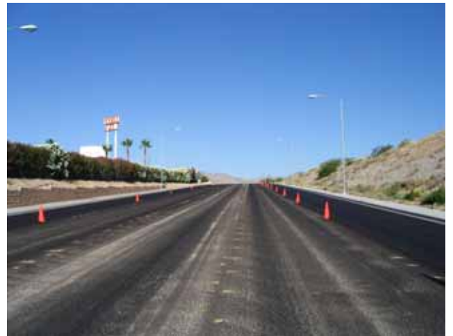
6. Sanding application by Clark County was applied at 2 lbs. sq. yard. (1 kg.sq. m.) A Spinner pull trailer was used.
