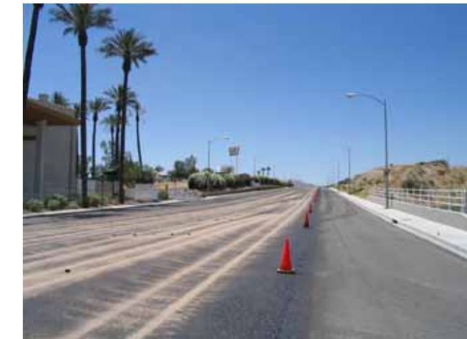
5. View of Civic Drive from Casino Drive. Outer lanes were coned off and traffic diverted to center lanes while outer lanes cured
